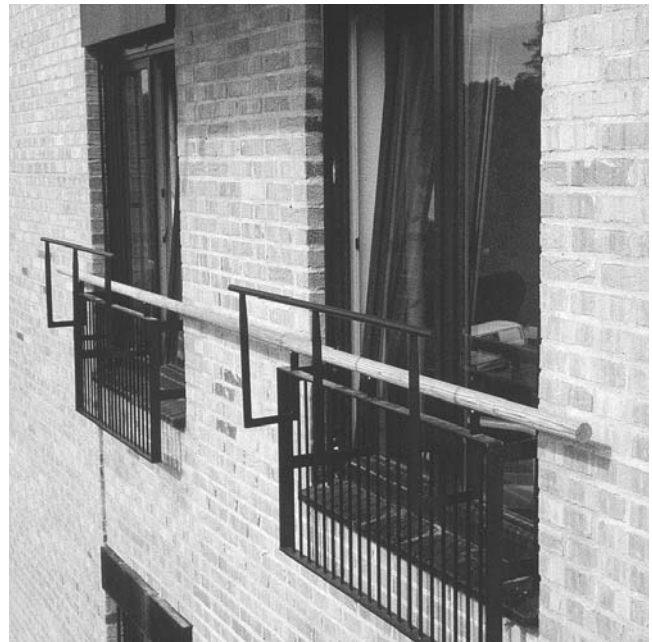
French balcony design is simple but elegant: This window grill design for the Bydel Søndre Nordstrand service house in Oslo, Norway, allows residents to place plants outside. The wooden dowel provides security and creates a two-window composition.
