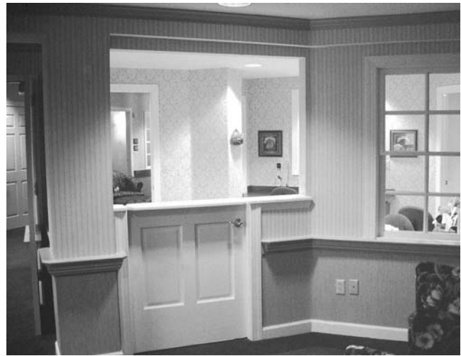
Dutch door is used to make nurse's office more approachable: This dementia office uses a fixed-pane glass window and a Dutch door to facilitate interaction between staff, residents, and family members at the Sunrise at Severna Park , Maryland.
